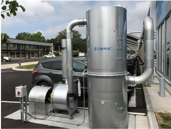
*Eurovac III System 10HP - 75HP Turbine Vacuum Producers and Bag Filter Separators*
