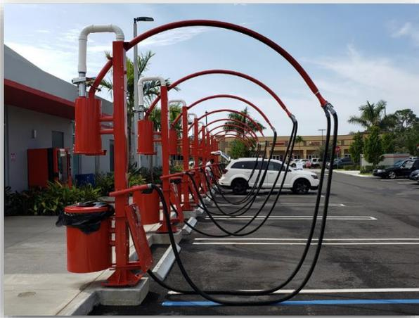
9' Curved Arches provide a uniform appearance as you look down the row of vacuum stalls. Arches come standard with a stainless steel interceptor that will separate the majority of material right after the arch. This helps reduce the risk of clogs within the central piping system.
